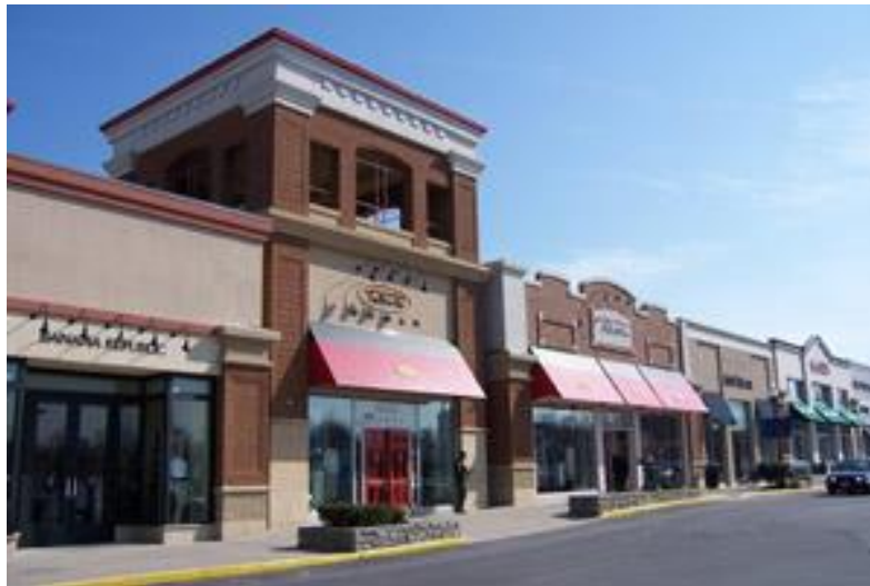
Figure 1210-E: Illustration of façade treatments such as pilasters, projections, and material changes to provide a visual façade offset.
