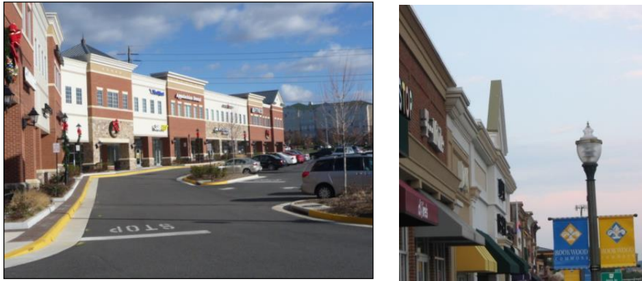
Figure 1210-G: Parapet walls with cornice treatments are used to disguise flat roofs. The image on the right illustrates a tall, thin parapet wall that is prohibited.
