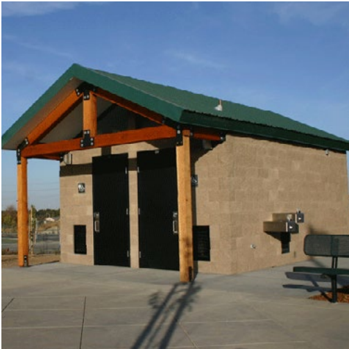
Restroom (Alt. 3) Manufacturer: Romtec Model: 2022 - Double Restroom Design: 2-single occupant, mechanical Color/Material: Coordinate with preferred shelter and site furnishing standards. Size: 12'8" x 16'8" (no porch), 17'8" x 16'8" (with 5' concrete walk/porch) Cost: $55k - 90k (design, material) + $82.5k - 135k (install)
