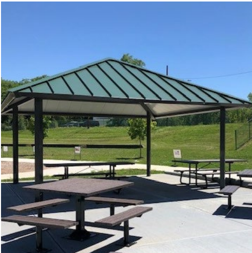
Shelter (Sunset) Manufacturer: Poligon Product: Square 20 Shelter Model: SQR-20 Color: Frame - Slate Gray; Roof - Evergreen Design: 20'x20'; SS (structural seam roof) Roof Pitch: 6:12 Cost: $31.4k (includes installation) Capacity: 6 picnic tables
