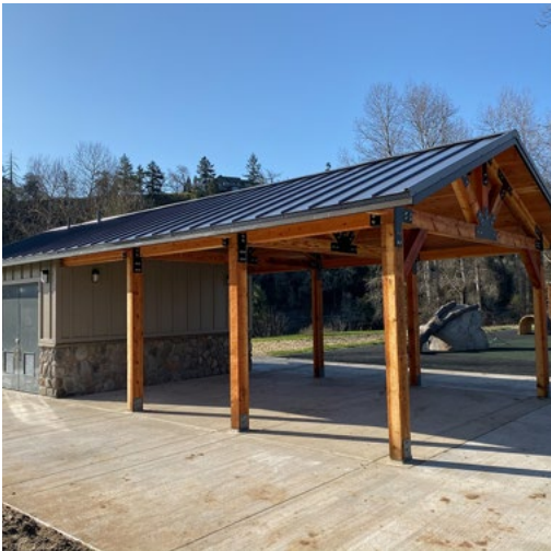
Restroom Upgrade (Attached Shelter) Manufacturer: Romtec Model: 20' Picnic Shelter Addition Color/Material: Coordinate with preferred shelter and site furnishing standards. Size: 27'4" x 16'8" Cost: $30k - 50k (design, material) + $30k - 50k (install)
