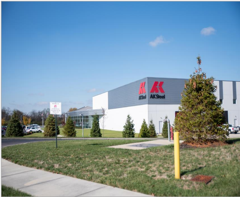
AK Steel Research & Innovation Center
