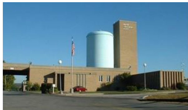
Water Treatment Plant
