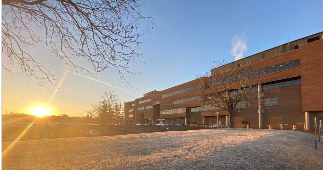
Middletown City Building facing southeast
