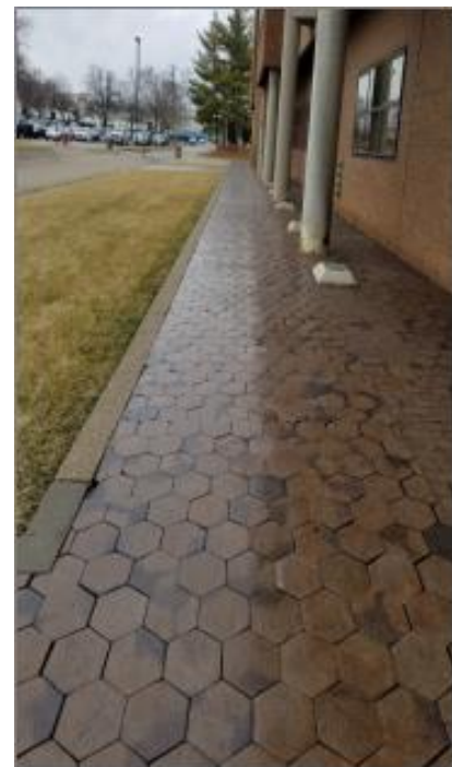
Plaza walkway pavers currently in use
