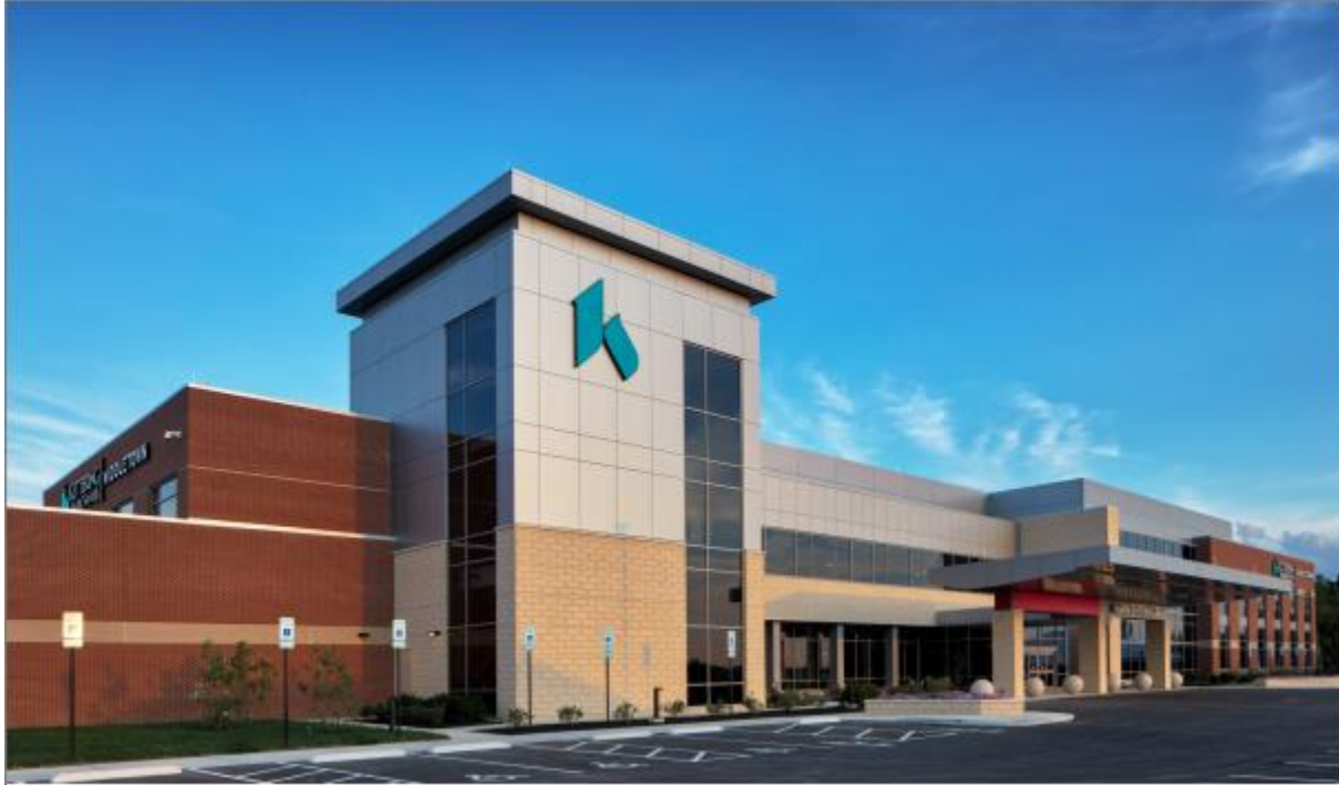
Kettering Health Network – Middletown, Ohio
