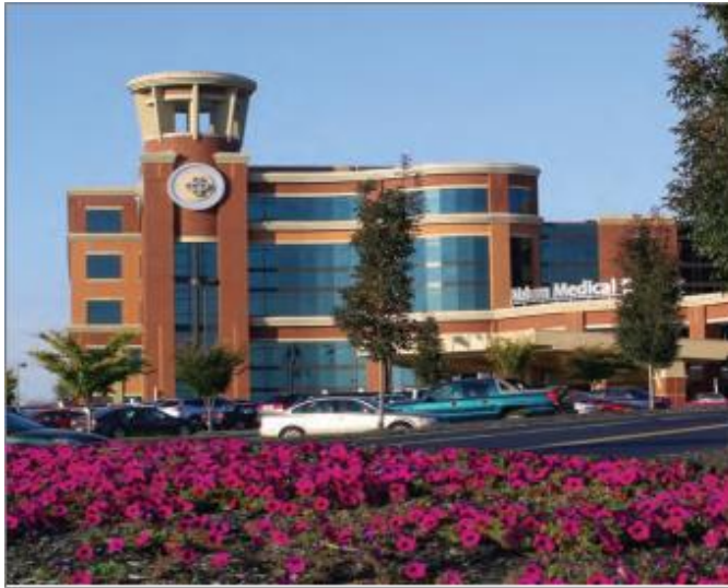
Atrium Medical Center on Premier Health Campus
