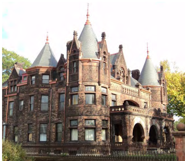
Photo of the Sorg Mansion
