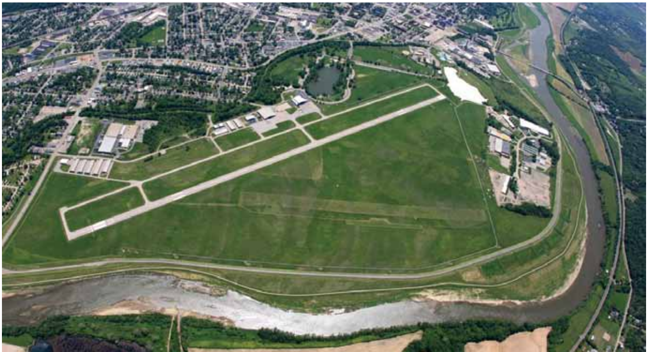
Middletown Regional Airport.
